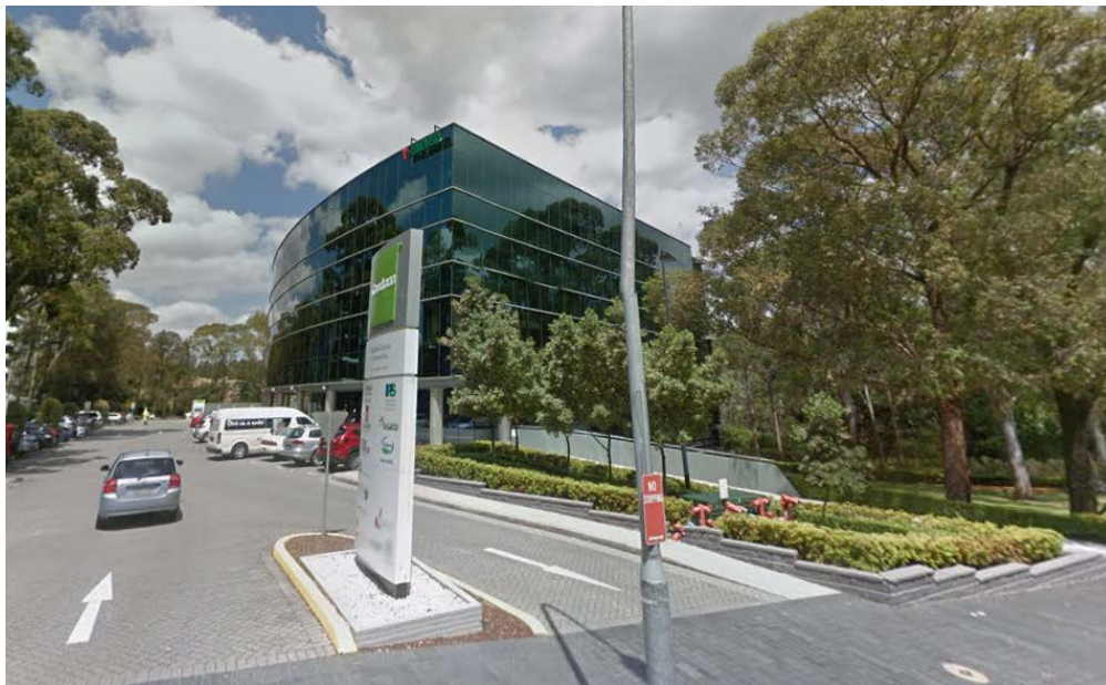
Figure 5: Existing building at 82 Waterloo Road to be demolish with recent approved for a mixed use development comprising of 2 x 20 storey mixed use buildings (Panel Reference 2017SNH009).
