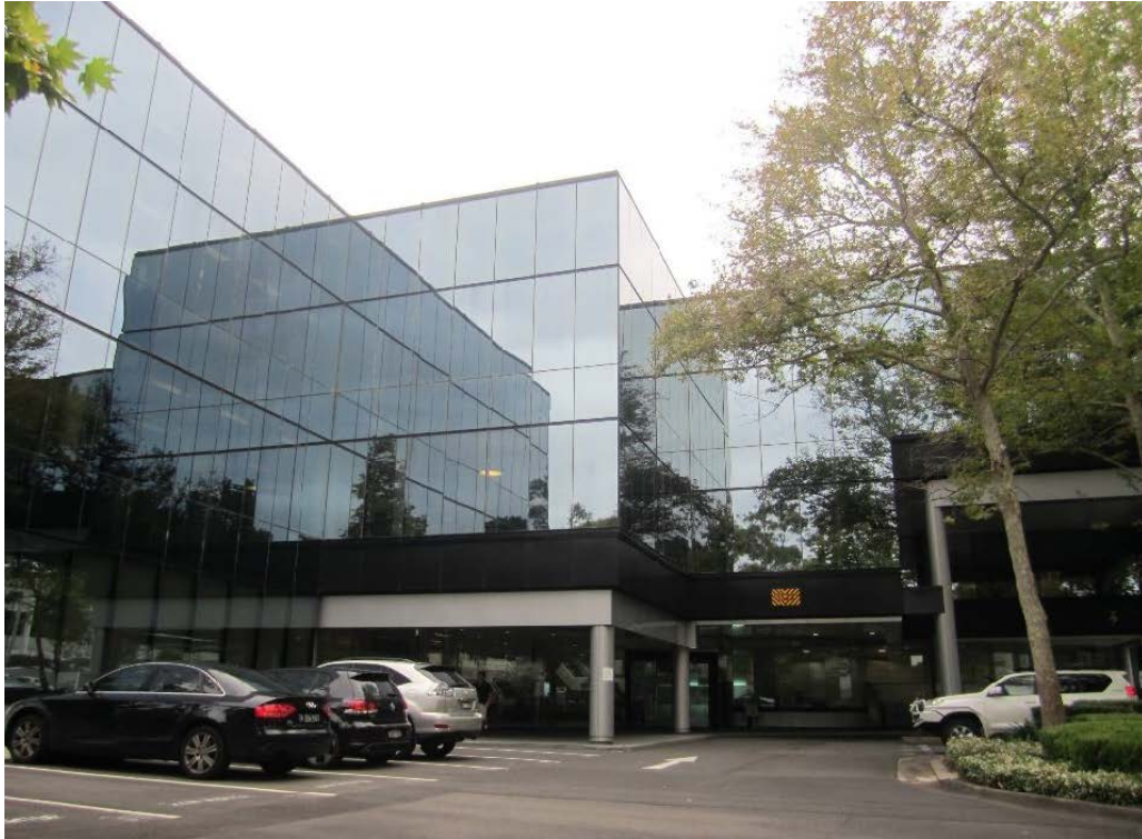
Figure 6: Existing building at 101-107 Waterloo Road to be demolish with recent approval for a mixed use development for 4 towers with a total rise of 23 storeys over a shared two storey podium. (Panel Reference 2017SNH010).
